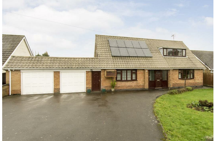
Double Garage 21'5" x 20'8" (6.53m x 6.30m)
